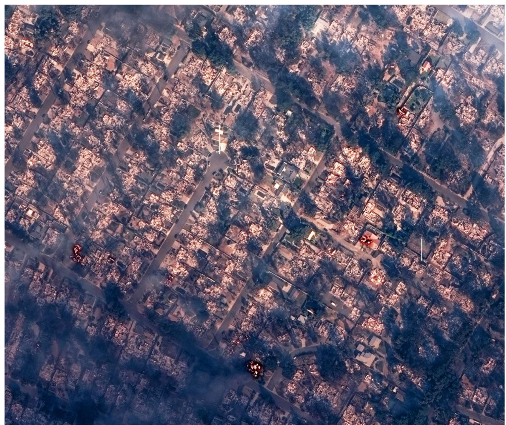
Example of Destruction Caused by Eaton Fire – Photo via Maxar Technologies
