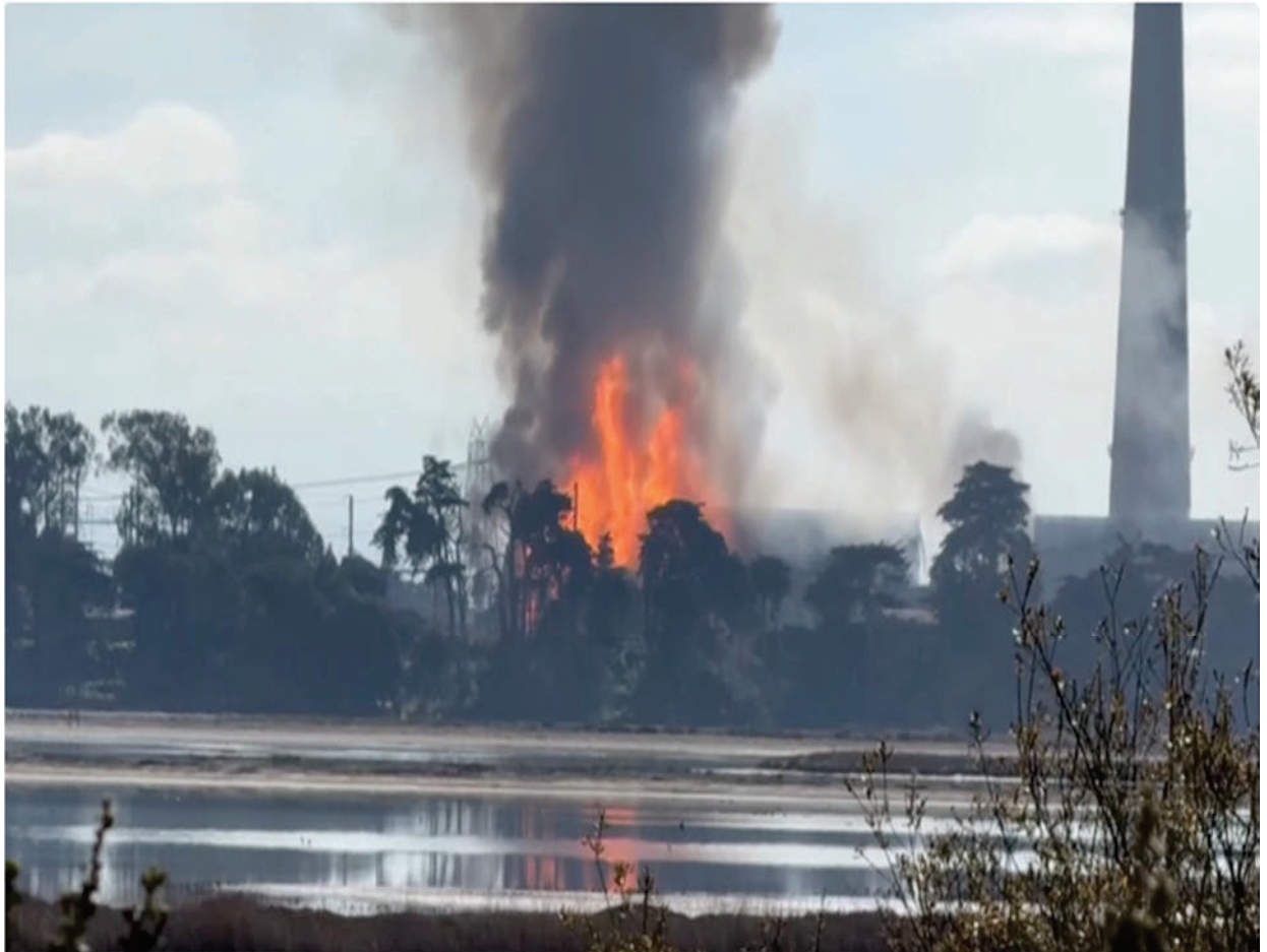
Figure 3 – Moss Landing Lithium Battery Facility Fire 5
